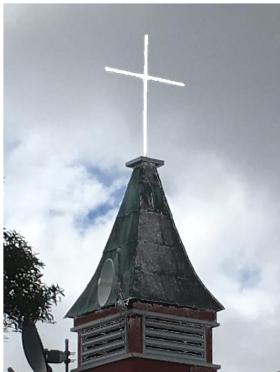
New cross added to the steeple.
