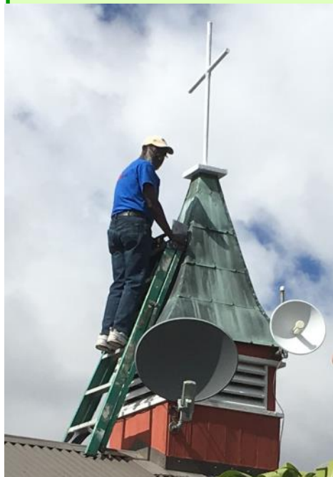
Steve polishes the new cross on the church steeple.
