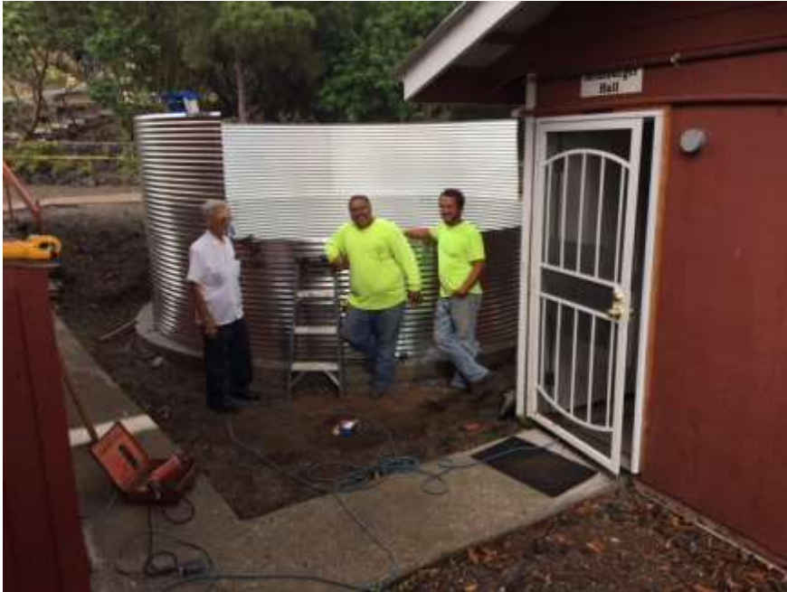
The new water tank was installed by Taylor Construction.
